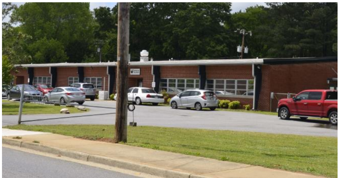
Figure 37. Bannon Hall, current image from survey.
