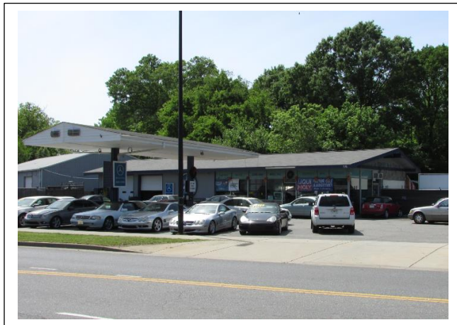
Figure 43. Pete's Super Gas Station (#4523), current image from survey.
