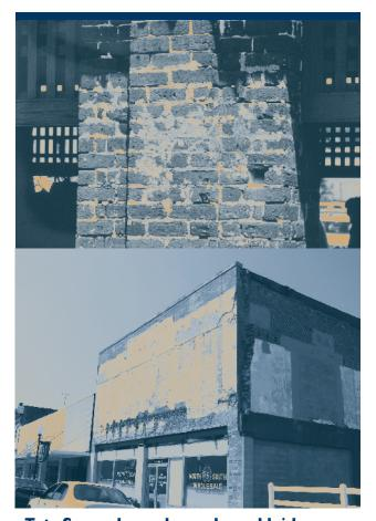
Top Several poorly made and laid mortar patches result in damage to the brick and a sloppy appearance.
