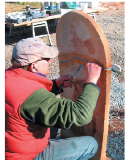
Figure 10: 0001.01, applying Repair Mortar
