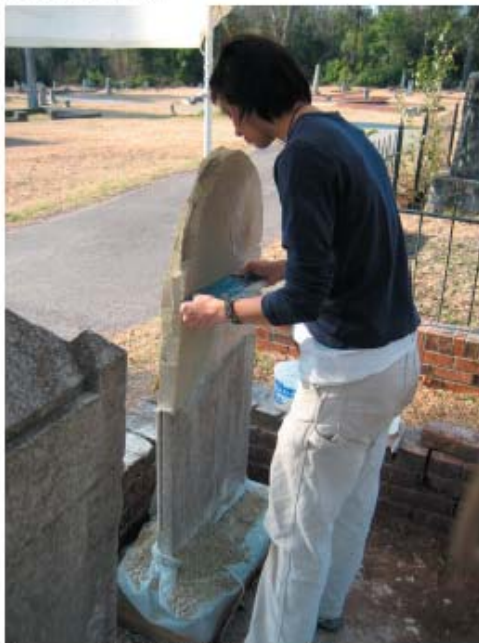
Figure 147: 0551.01, screeding repair mortar
