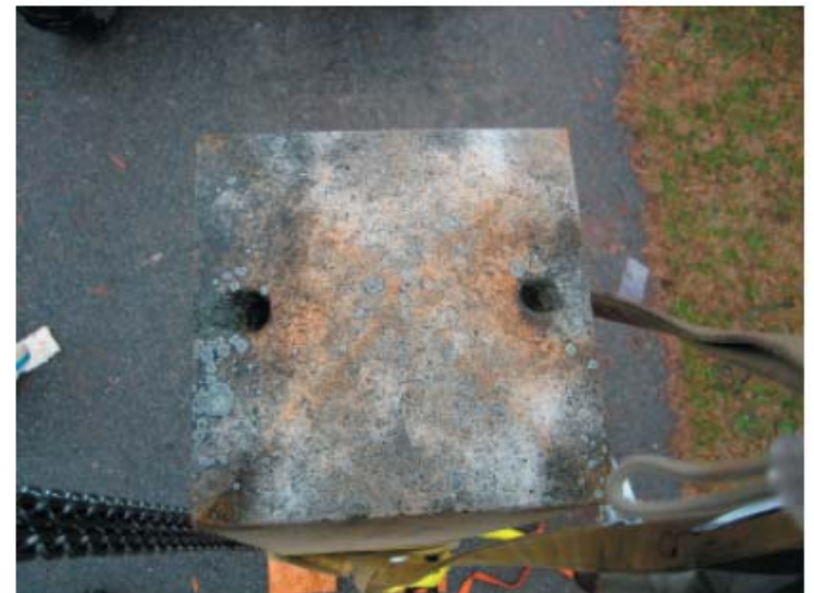
Figure 202: 0692, Lewis Pin holes in top of obelisk
