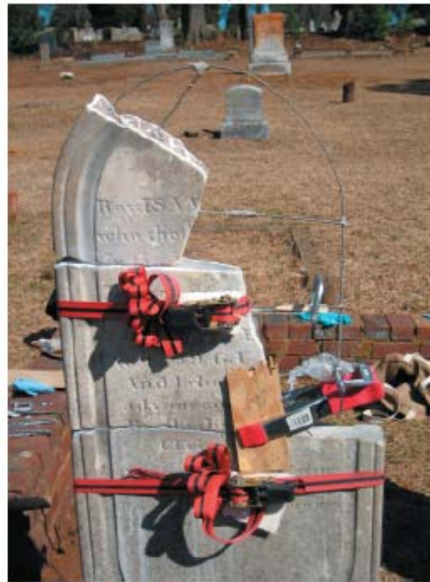
Figure 146: 0551.01, tablet reassembled
