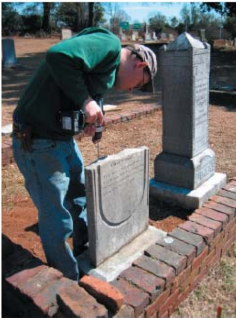
Figure 145: 0551.01, drilling pin holes into the tablet
