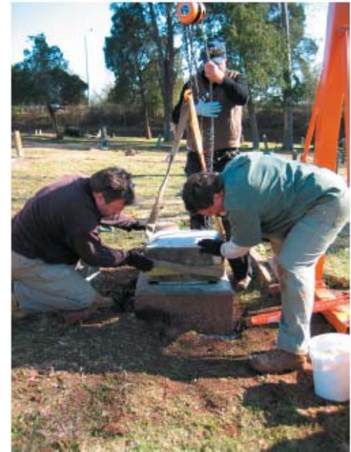
Figure 36: 0101, reattaching the plinth
