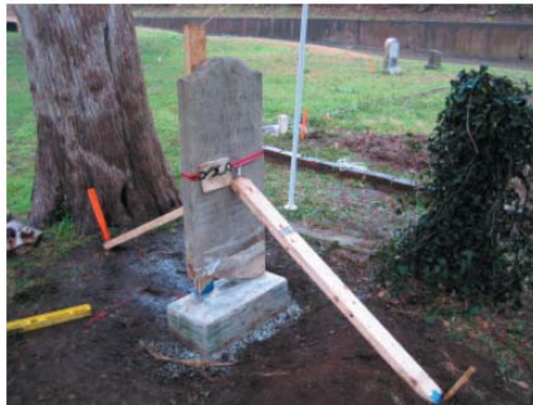
Figure 69: 0112.06, tablet reinstalled
