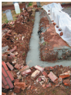
Figure 7: 0001.01, new foundation poured
