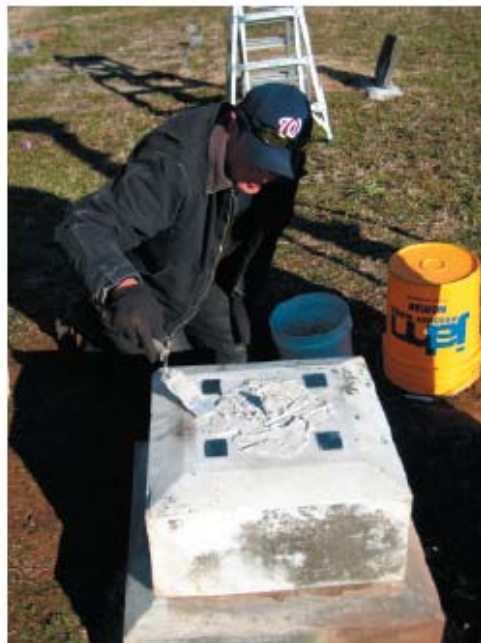
Figure 37: 0101, preparing to reattach the pillar
