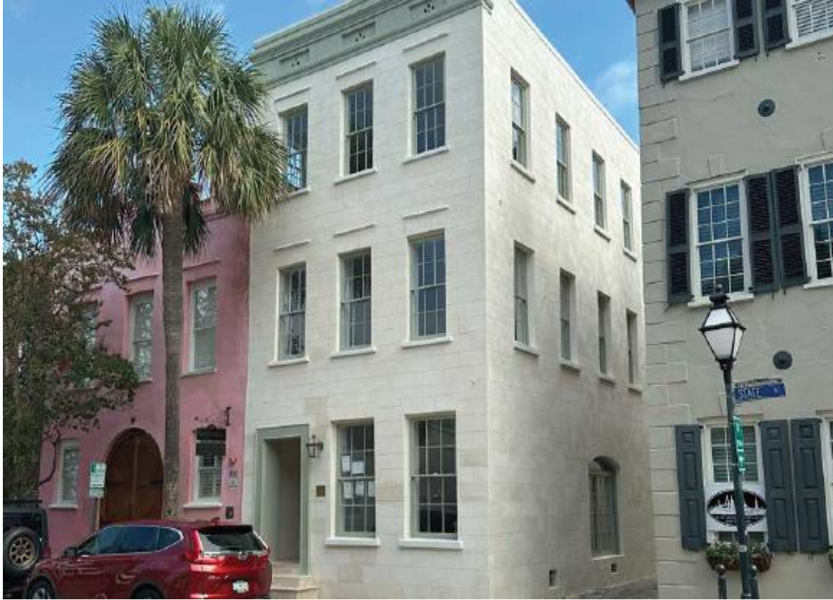
After rehabilitation photo of the c. 1799 residence at 44 State Street in Charleston
