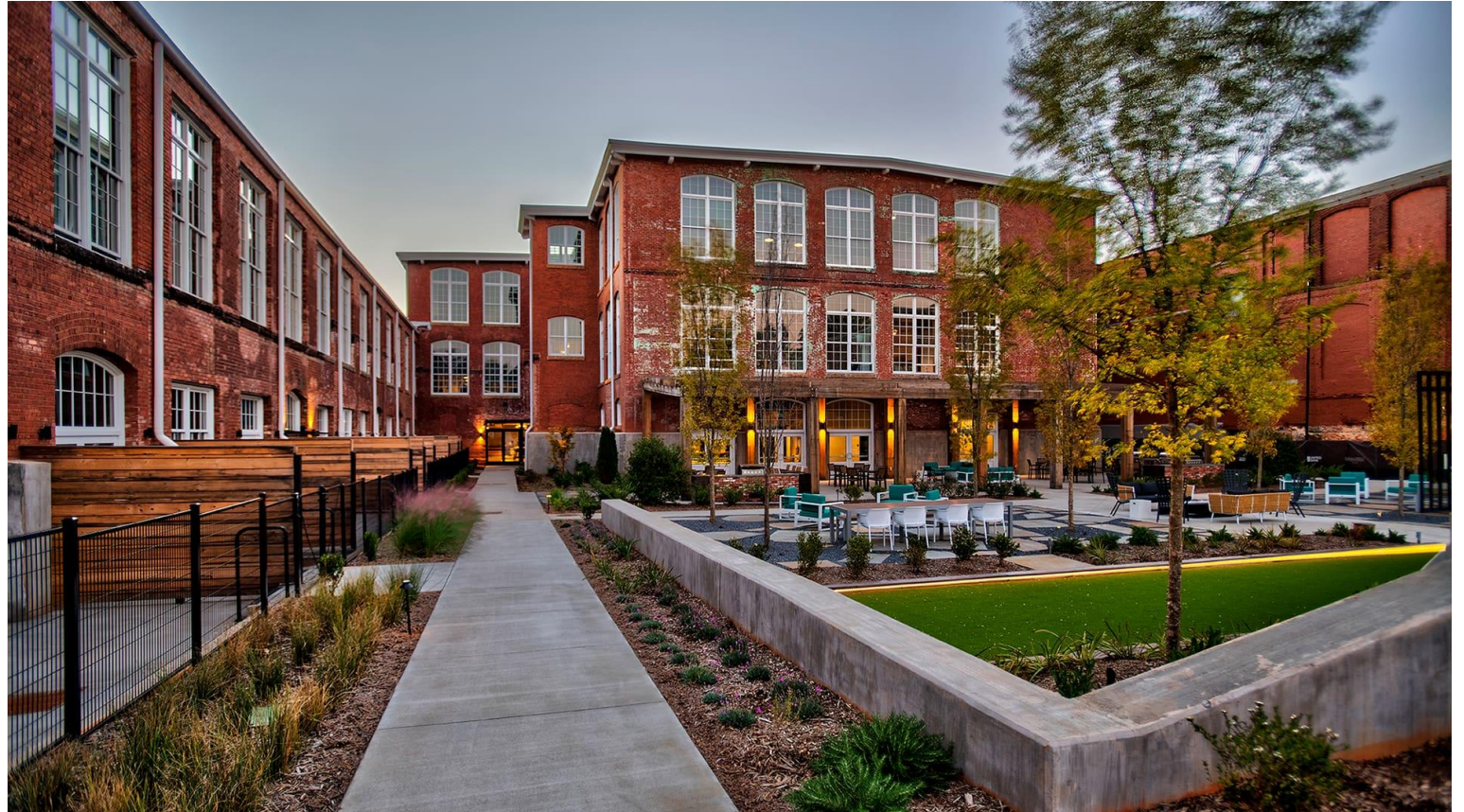
After rehabilitation photo of the historic Judson Mill
