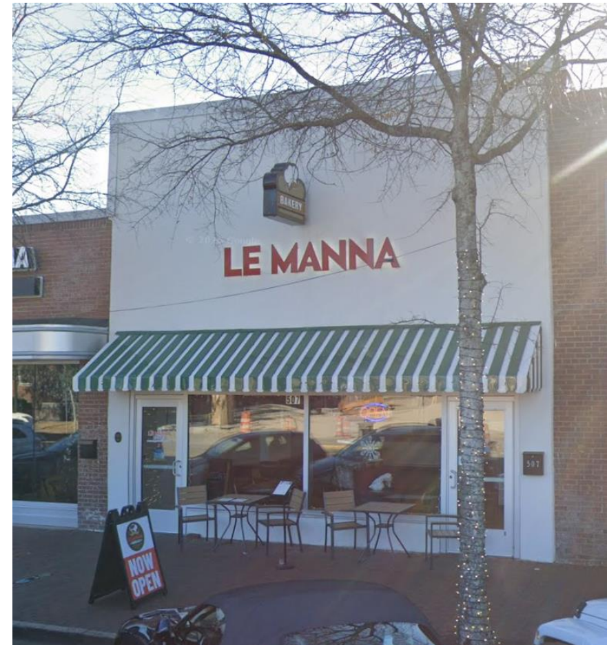
After rehabilitation photo of the historic c. 1946 bakery commercial building at 509 9 th Avenue in Myrtle Beach
