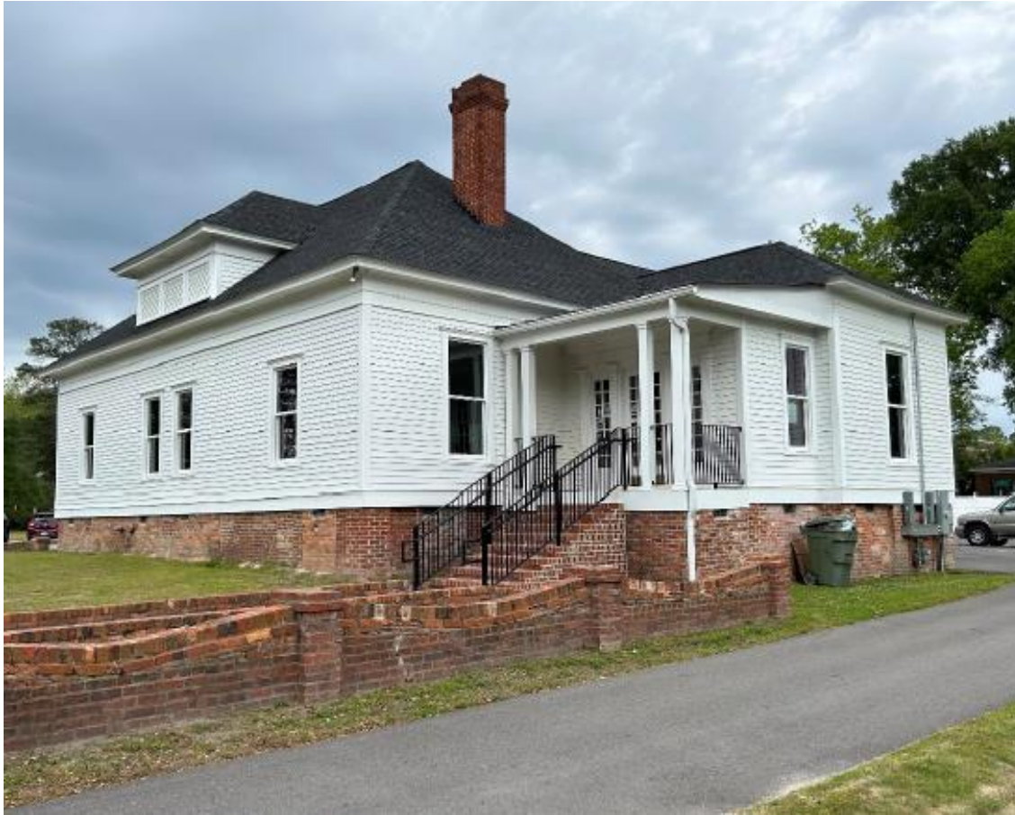
After rehabilitation photo of the historic c. 1902 residence at 310 Hampton Park in Camden
