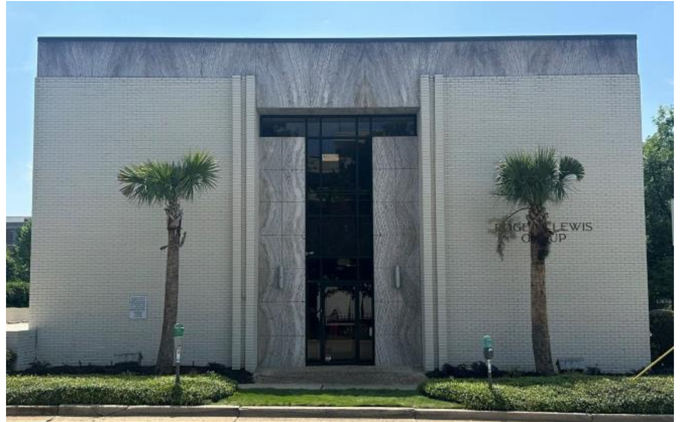
After rehabilitation photo of the historic Bob Russell Realty Offices
