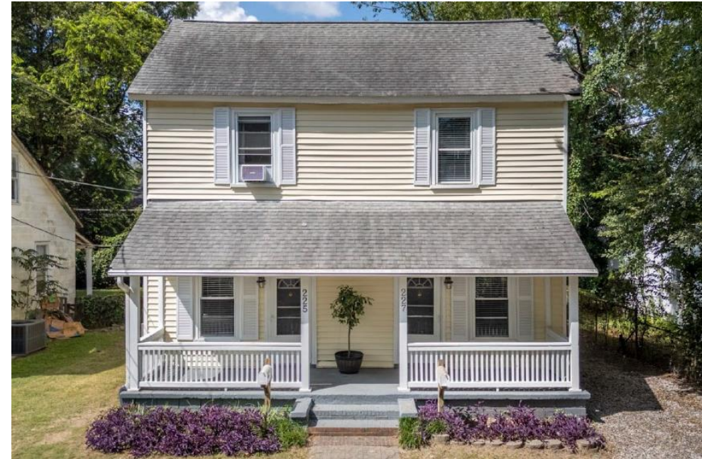
After rehabilitation photo of the historic c. 1900 mill duplex at 225 Tryon Street in Columbia's Granby Mill Village Historic District
