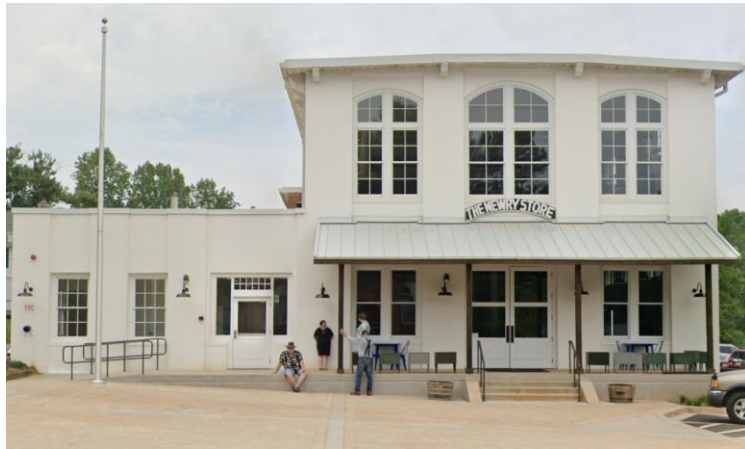
After rehabilitation photo of the historic c. 1894 Newry Mill Store and Post Office
