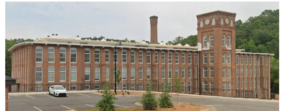
After rehabilitation photo of the historic c. 1893 Courtenay (Newry) Mill
