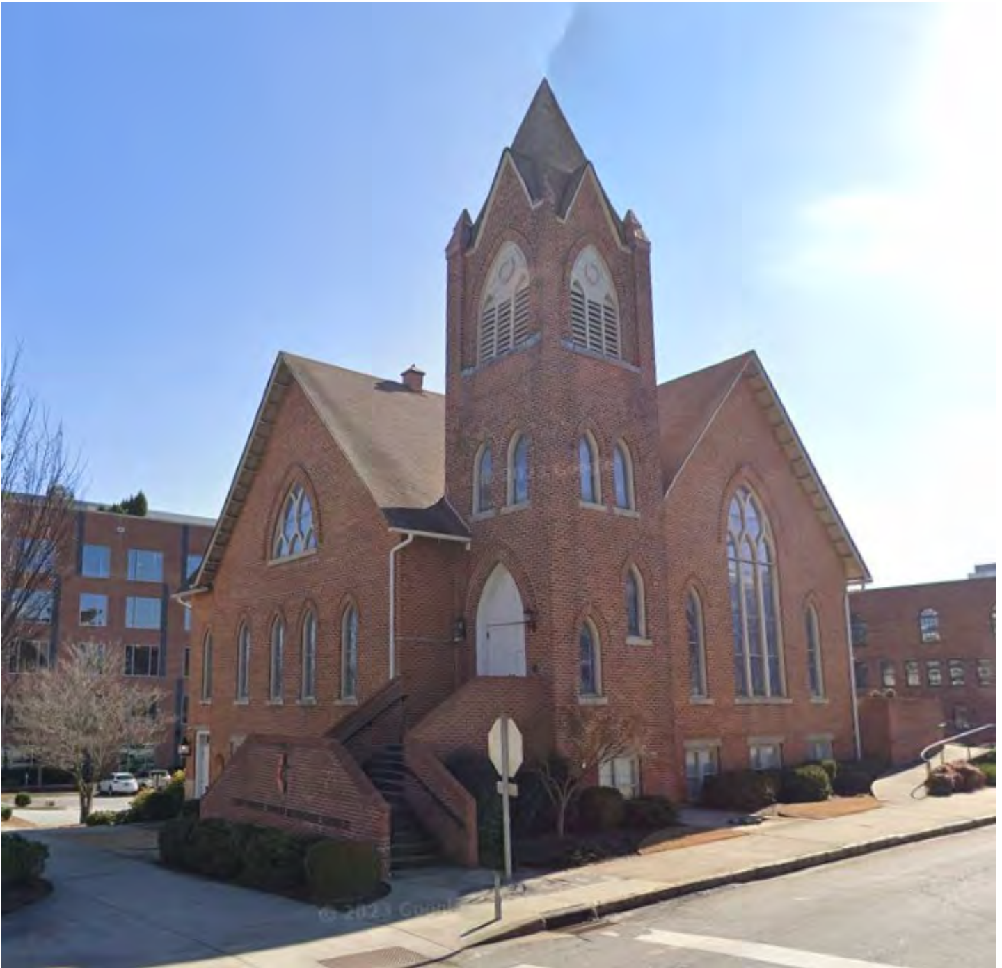
Figure 13. John Wesley United Methodist Church (100 Court Street), a historically African American congregation, built a new church between 1900-1903 in the Gothic Revival style, shown here. Image by Google Street View, 2023.
