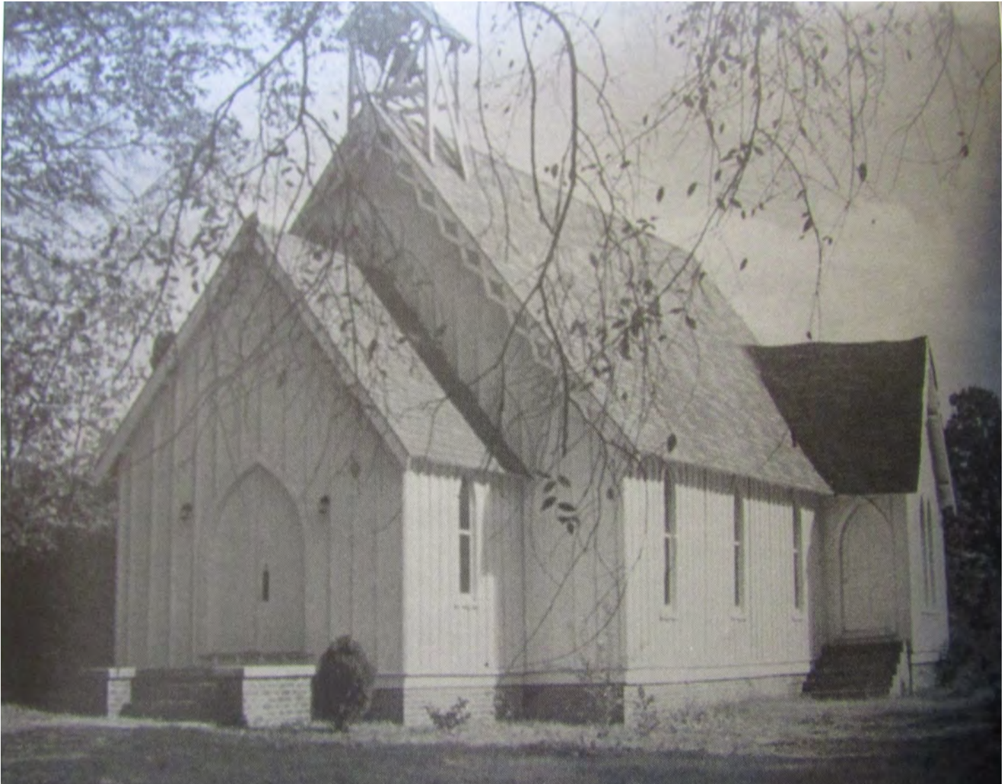
Figure 11. Christ Church in Lancaster, designed and built by John D. McCollough, completed in 1882 (not extant). Note the decorative bargeboard in the front gable of this Carpenter Gothic style church. The shape of the building is very similar to St. Andrew's Episcopal Church. Image from the book Building the Walls of Jericho , John DeWitt McCollough and His Churches, Judith Bainbridge, no page number.
