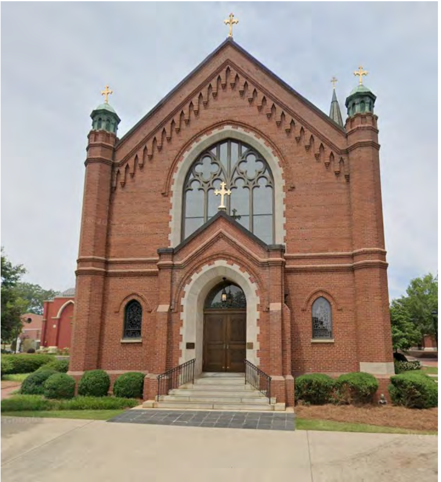
Figure 12. St. Mary's Catholic Church (Greenville) was completed in 1904 and features a repeated brick corbel detail framing the front gable, a detail also found on St. Andrew's Episcopal Church, completed in 1905. Image by Google Street View, 2023.
