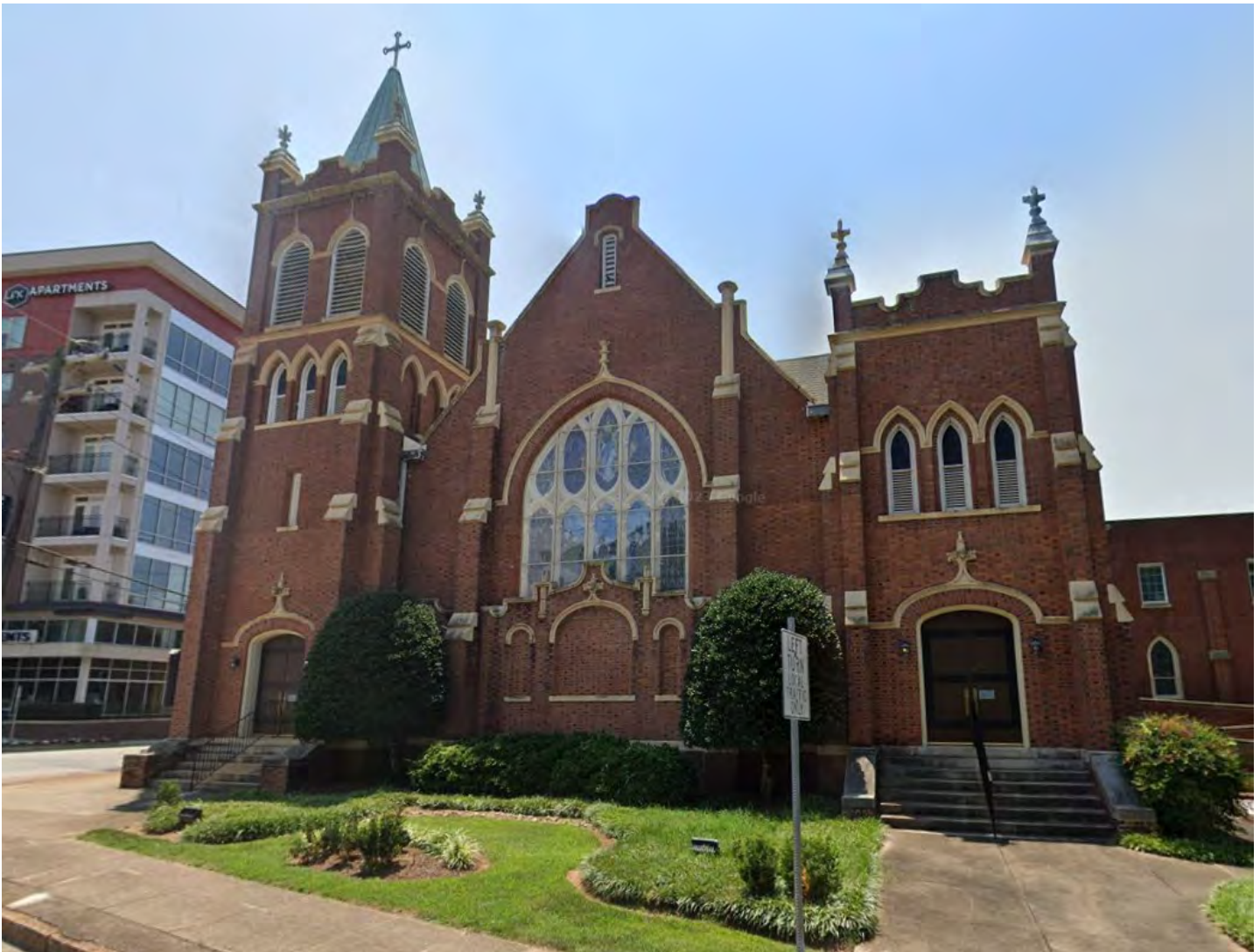
Figure 15. Second Presbyterian Church in Greenville, completed in 1909, is a higher style Gothic Revival building than St. Andrew's Episcopal Church. Image by Google Street View, 2023.
