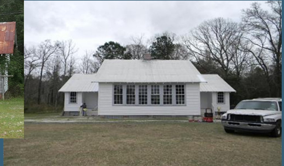
Bull Swamp Colored School Orangeburg County, March 2024. After stabilization.
