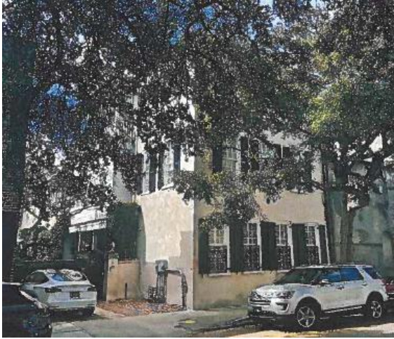
After rehabilitation exterior façade. Image courtesy of Meadors, Inc.
