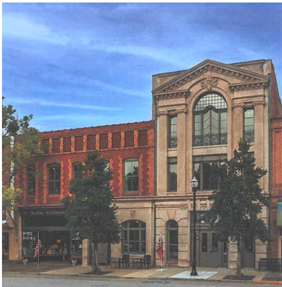
Photograph of the First National Bank of Camden after rehabilitation in 2021. Image courtesy of Scott Lambert.
