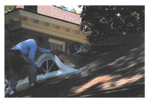
Workers replacing in-kind a severely deteriorated dormer window. Image courtesy of the applicants.
