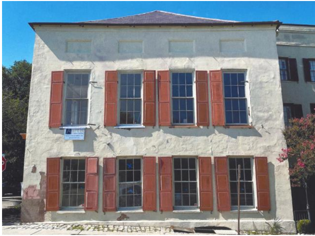
Pre-rehabilitation photograph of the wharf building. Image courtesy of Brittany Lavelle Tulla, 2020.
