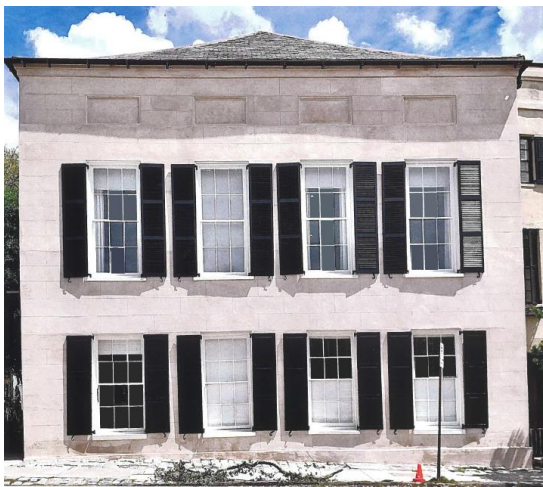
Post-rehabilitation photograph of the wharf building. Image courtesy of Brittany Lavelle Tulla, 2021.
