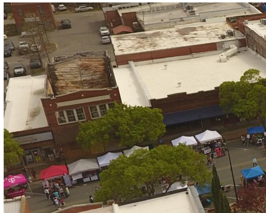
Collapsed roof at 153 Market Street
