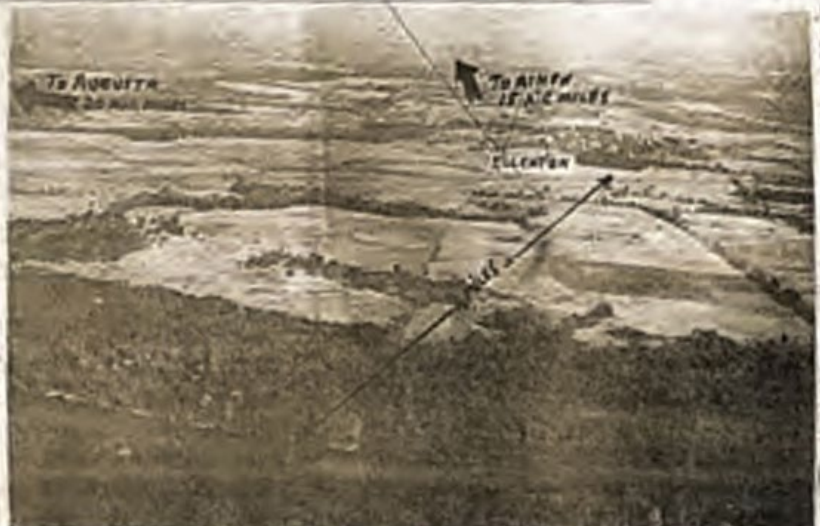
WHERE PORTION OF H-BOMBING FACILITY WILL BE LOCATED. The aerial photo shows what will probably be the heart of the big atomic energy production plant to be constructed on the 1,000-acre tract about 2 1/2 miles north of Augusta. Four miles in the construction cost of the huge project will be devoted to make way for the plant.
