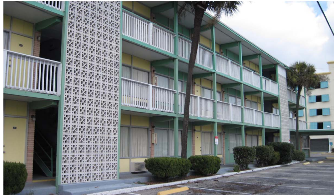
Concrete veil block on motel in Myrtle Beach (c.1965) Horry County Historic Resource Survey
