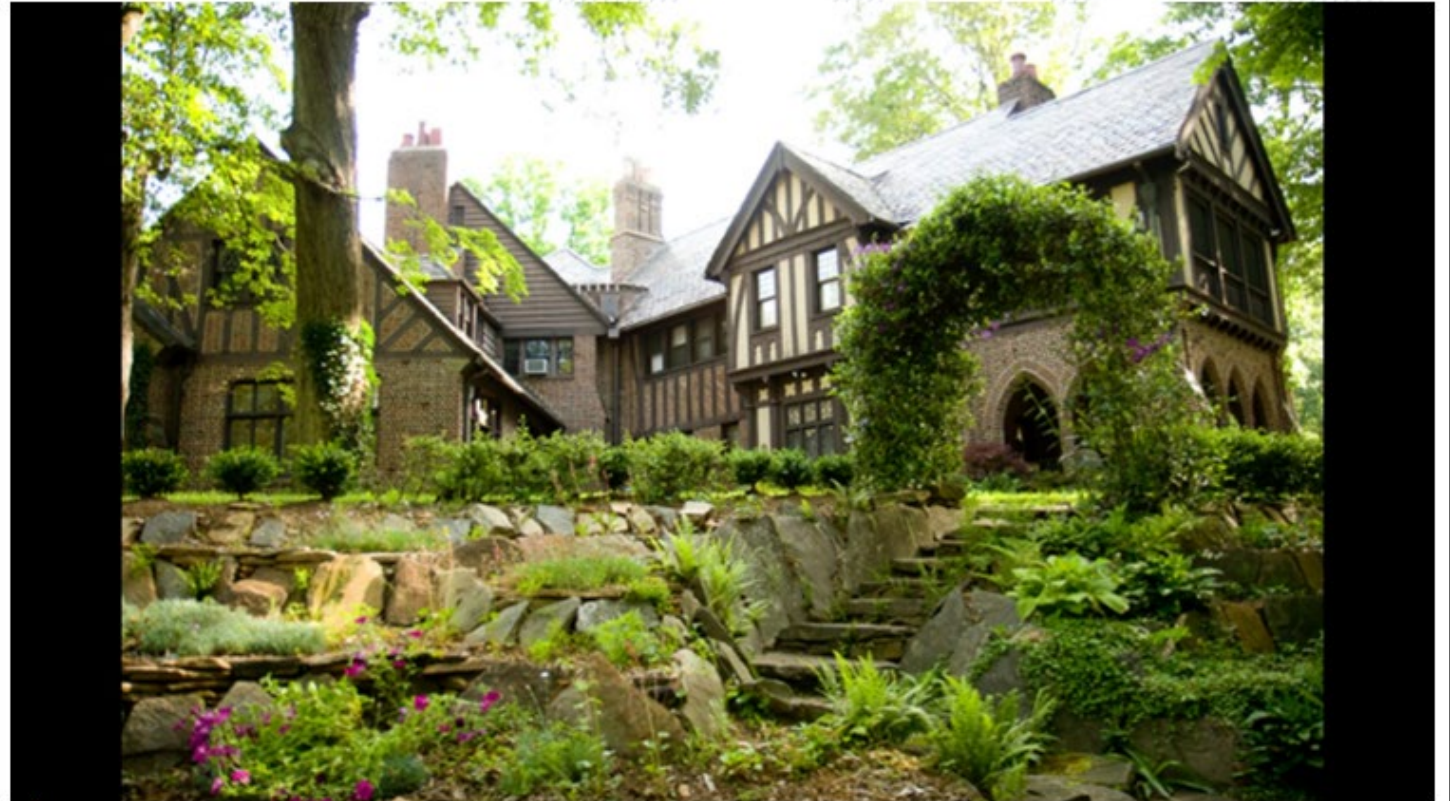
Demolition of Glenridge Hall could begin in a few days, despite a last-minute push to save it.
