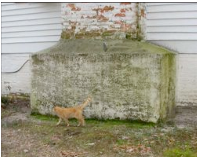
C. Replacement Chimney Base
