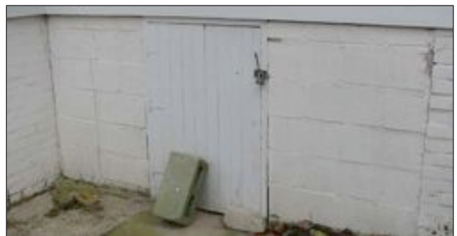
D. Concrete Block Foundation Infill and Crawlspace Door, Northeast Porch End
