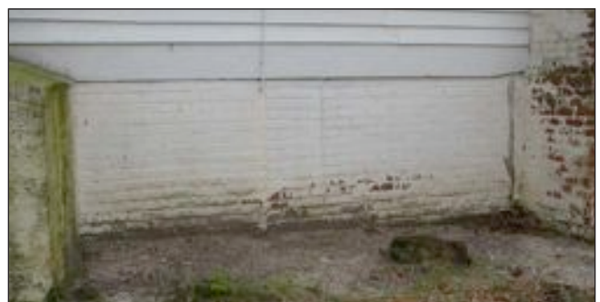
E. Brick Infill and Brick Pier Foundation, Northeast Porch End
