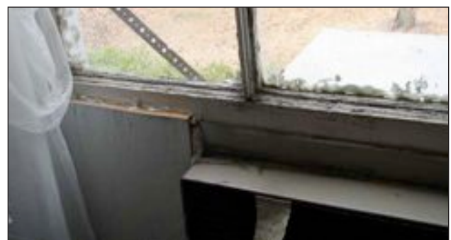
E. Paint and Possible Water Damage Around A/C Unit in Figure 16B
