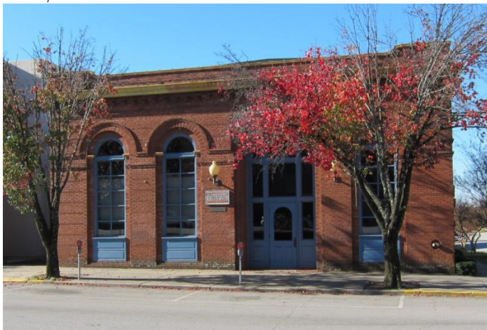
Photograph of the Columbia Electric Street Railway, Light & Power Substation after rehabilitation. Image courtesy of Swampfox Inc.
