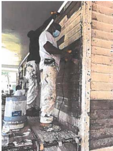
Photograph of the F.B. McBee House during rehabilitation. Image courtesy of Robert C. Benedict.
