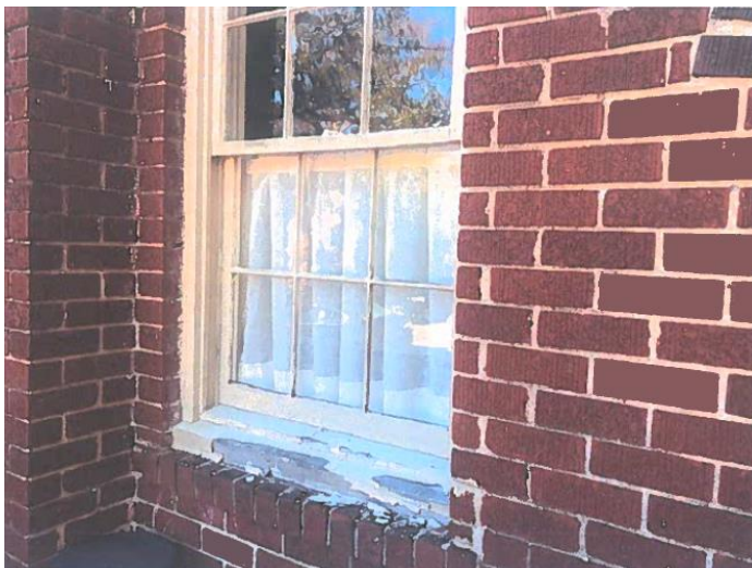
Before rehabilitation photograph, showing paint deterioration. Image courtesy of owner.
