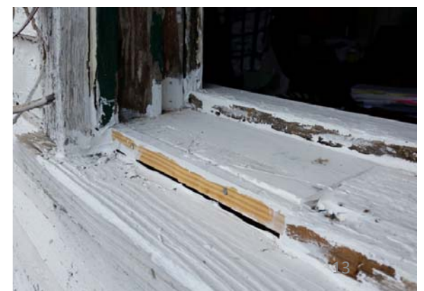
Bad repair to hole in sill causing water damage
