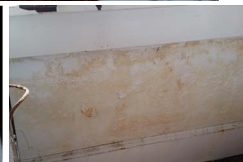
Bad repair to hole in sill causing water damage
