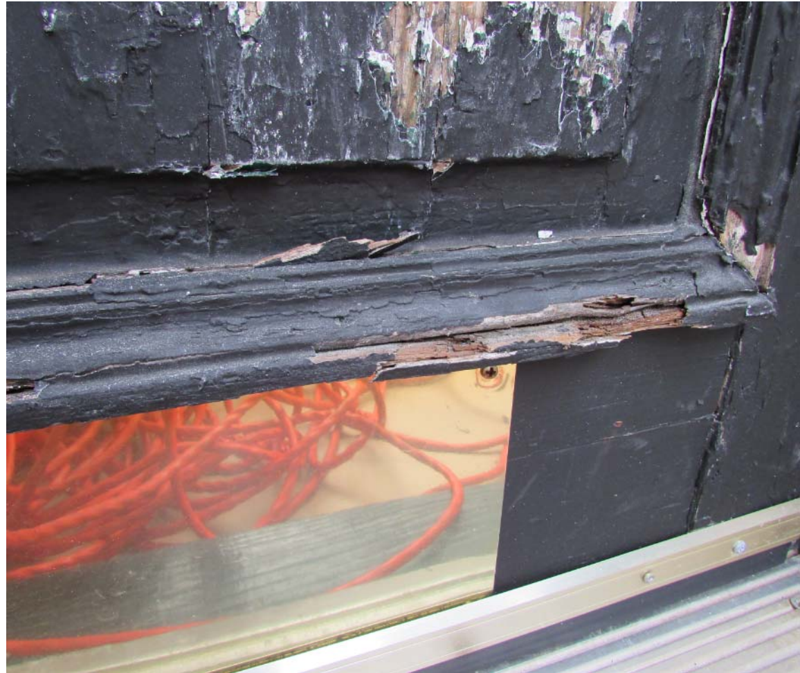
Door fully stripped (left) and problem area (above) repaired with wood hardener and epoxy
