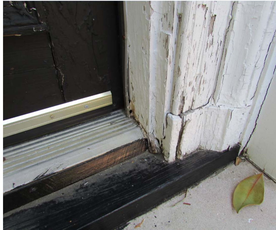
Used heat gun to remove old paint, had repairs to make from old water damage
