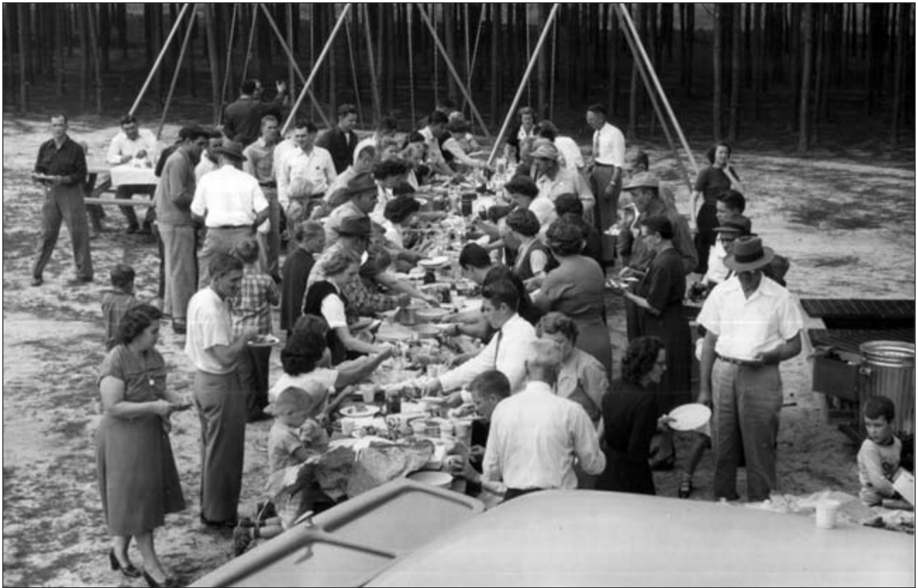
Central Shops Blacksmith's Bar-B-Que at Recreation Park No. 2.
