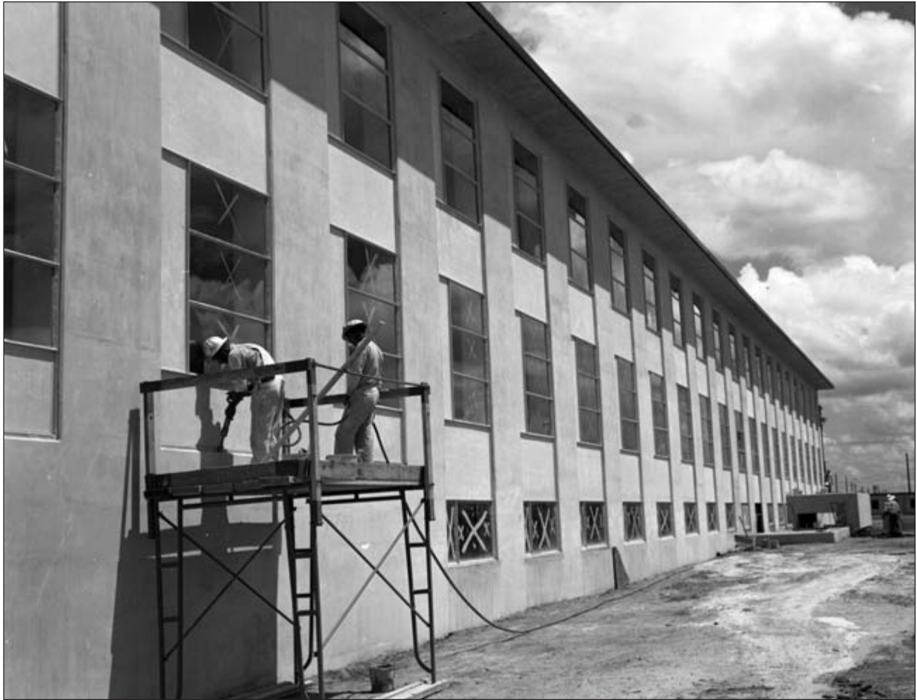
Construction workers put the finishing touches on Building 703-A, 1952.
