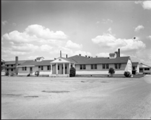
A. Atomic Energy Commission Building
