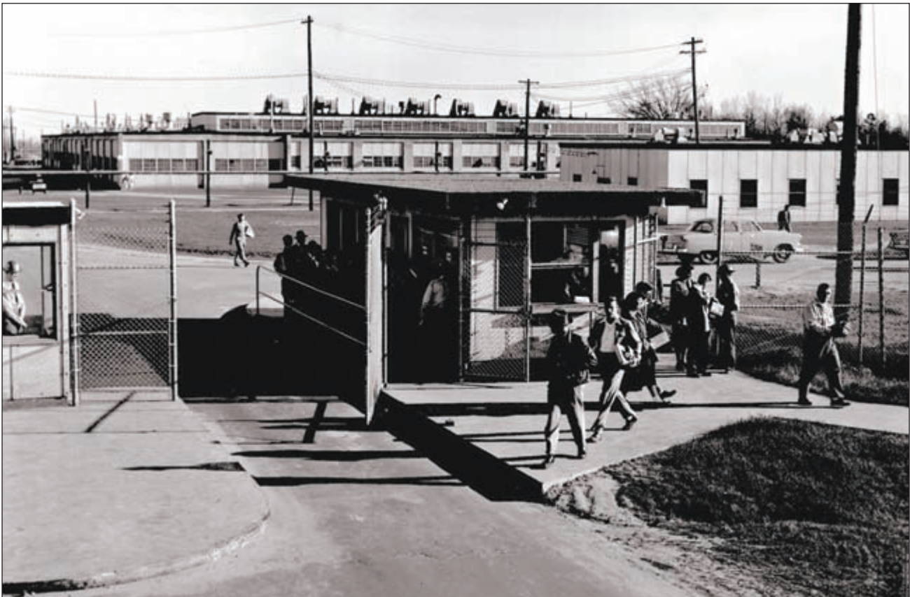
Employees passing into and out of a Limited Area, by way of the guardhouse.
